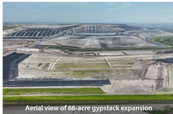
3-layer geosynthetic containment installation
